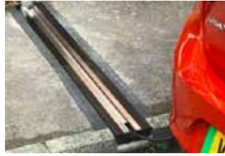
A pavement gully
